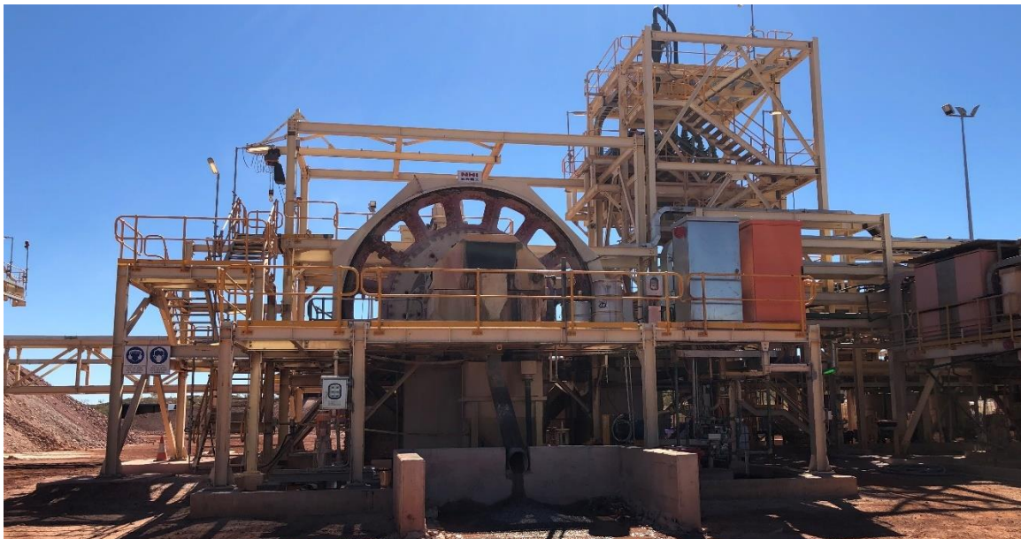
Figure 1: View of the Browns Range Pilot Plant beneficiation circuit
