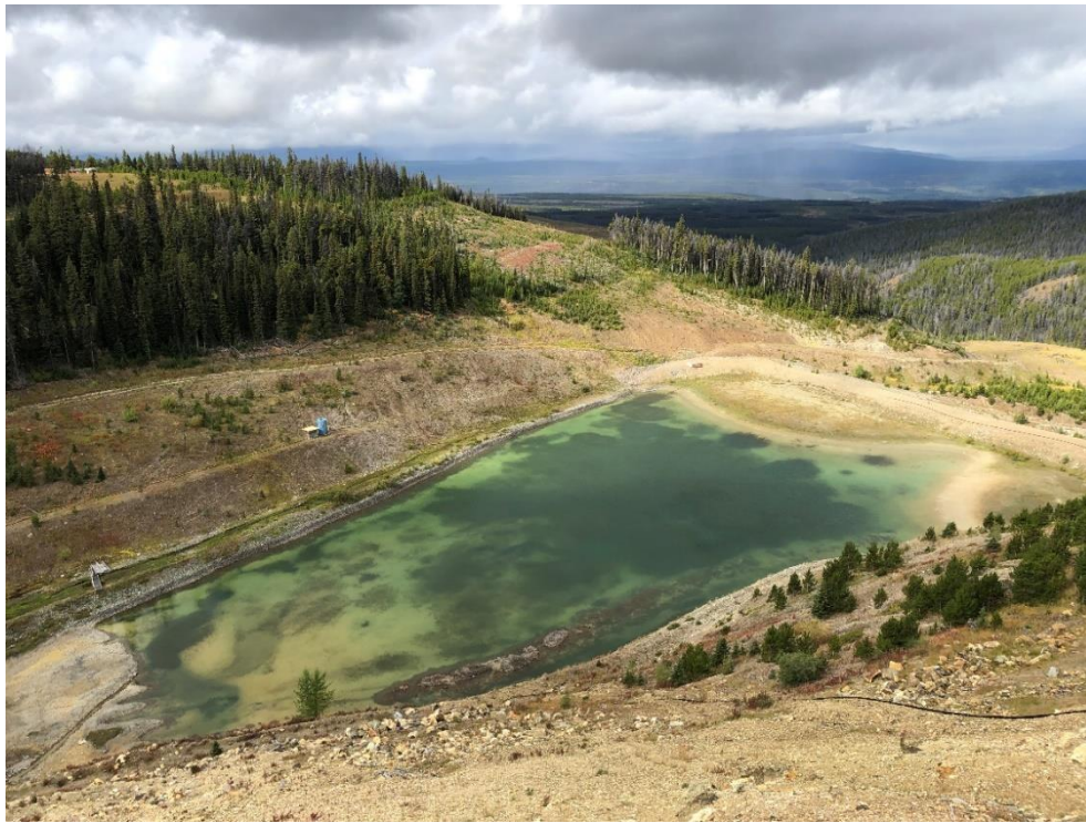
Figure 9 – Blackdome Tailings Storage Facility
