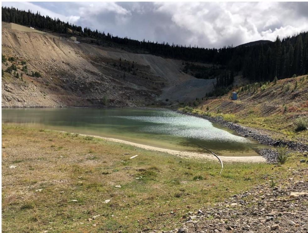
Figure 10 – Blackdome Tailings Storage Facility
