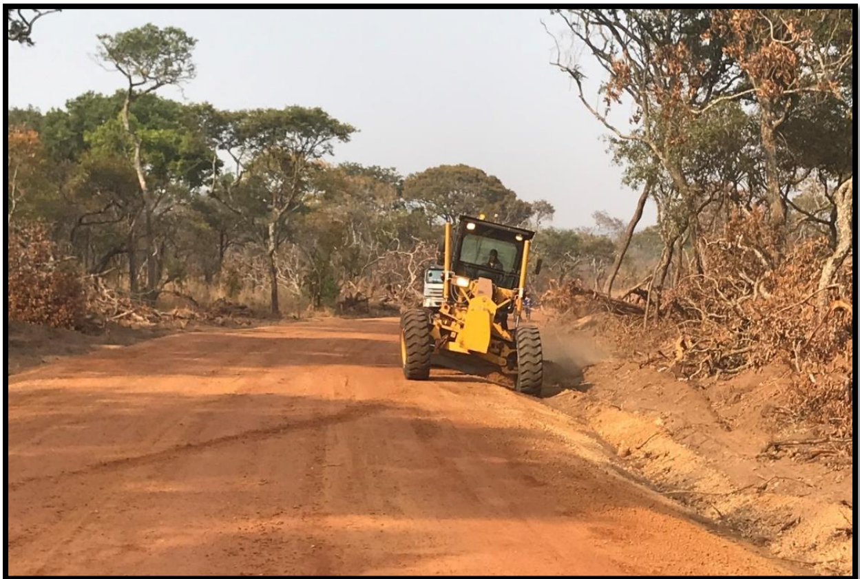
Final Grading of new road
