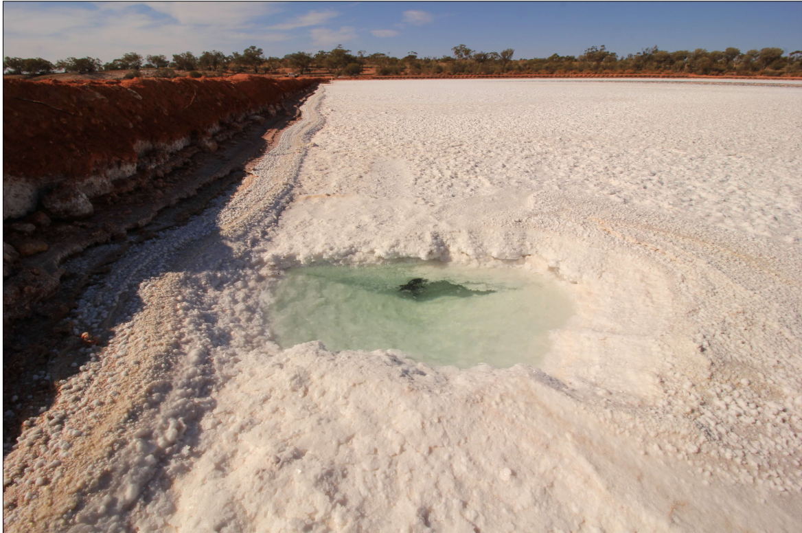
Figure 1: On-playa trial pre-concentration pond demonstrated low-cost, efficient lateral seepage barrier construction techniques using the highly stable and easily accessible playa perimeter
