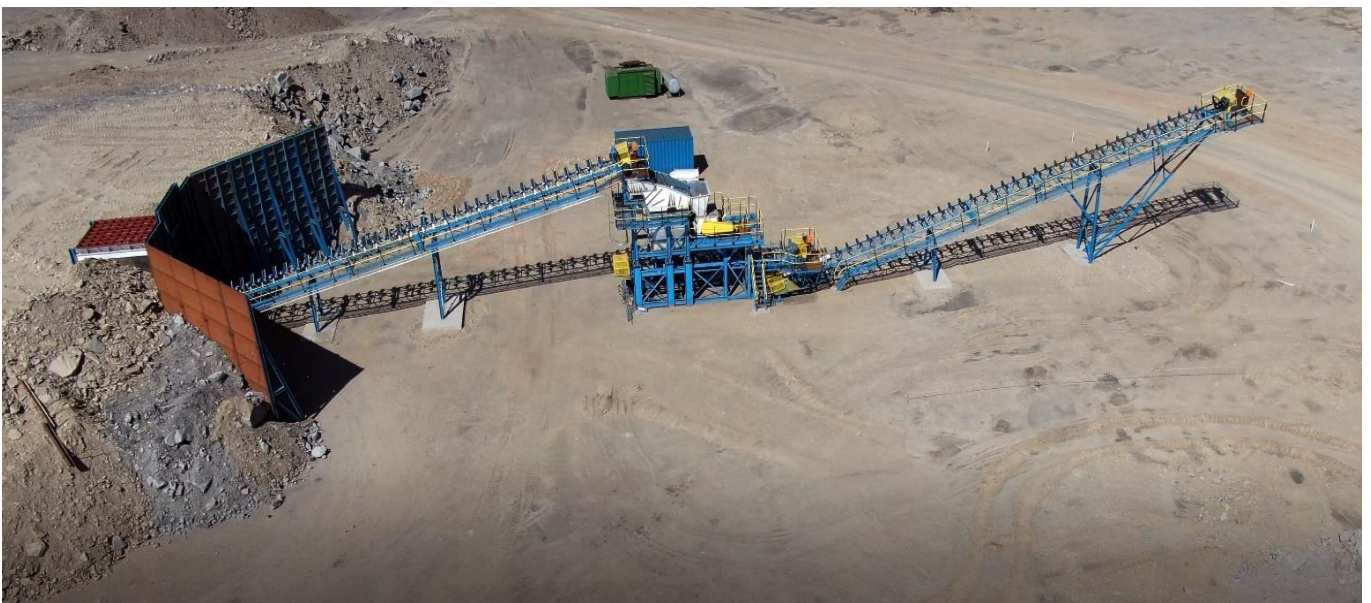
Newcastle project – Kliprand colliery - Installation of new crusher at the opencast area to replace rented moveable crushers currently being used in progress.
