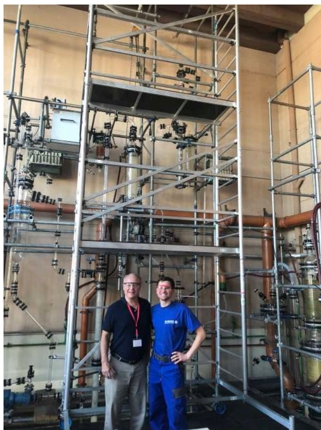
Figure 3: Bromine Pilot Plant Upper Floor
