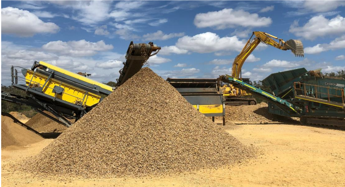
Figure 9: Crushing Infrastructure onsite at Far Fanning- crushing Low Grade Stockpiles
