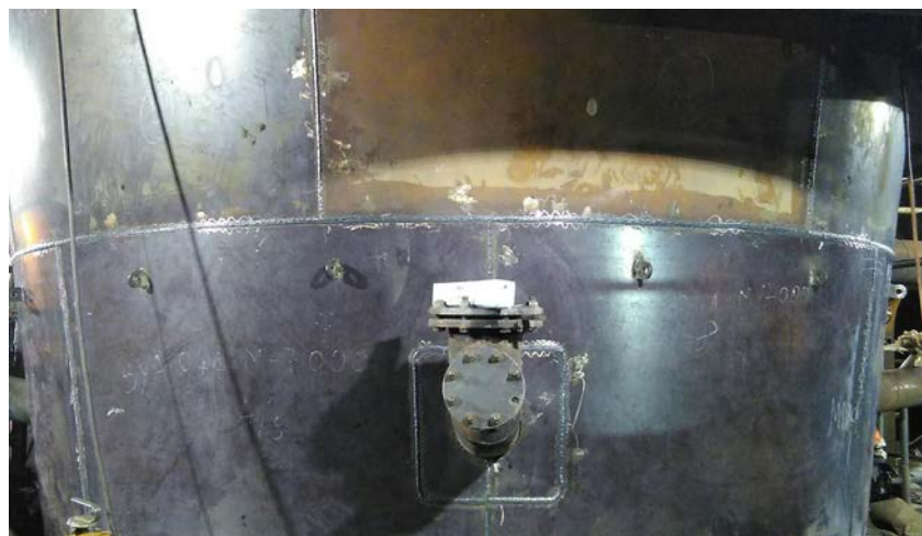
Figure 3: Photo showing progress of repairs to the Roaster. New plates have been welded to form a shell around the damaged area of the Roaster as depicted in Figure 2
