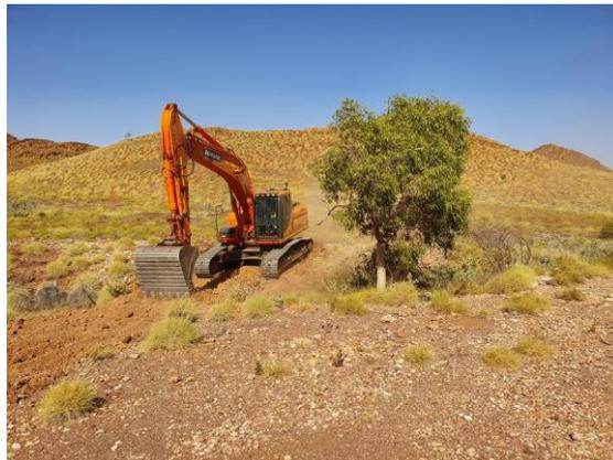
Fig 2 Grader and excavator preparing access and drill-pad at the Top Camp gold prospect on E47/2150.
