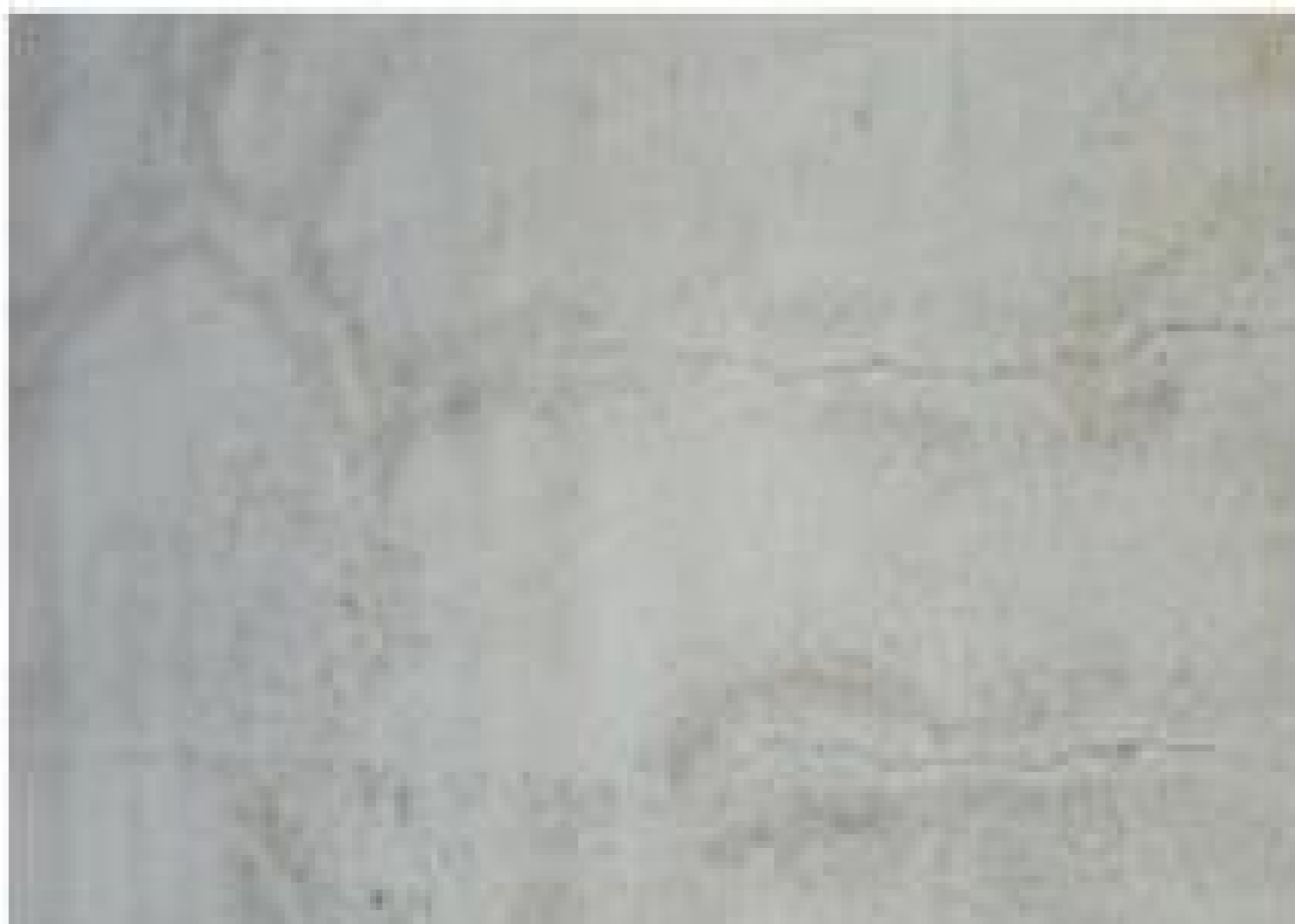
CONTROL TRIAL SLAB
