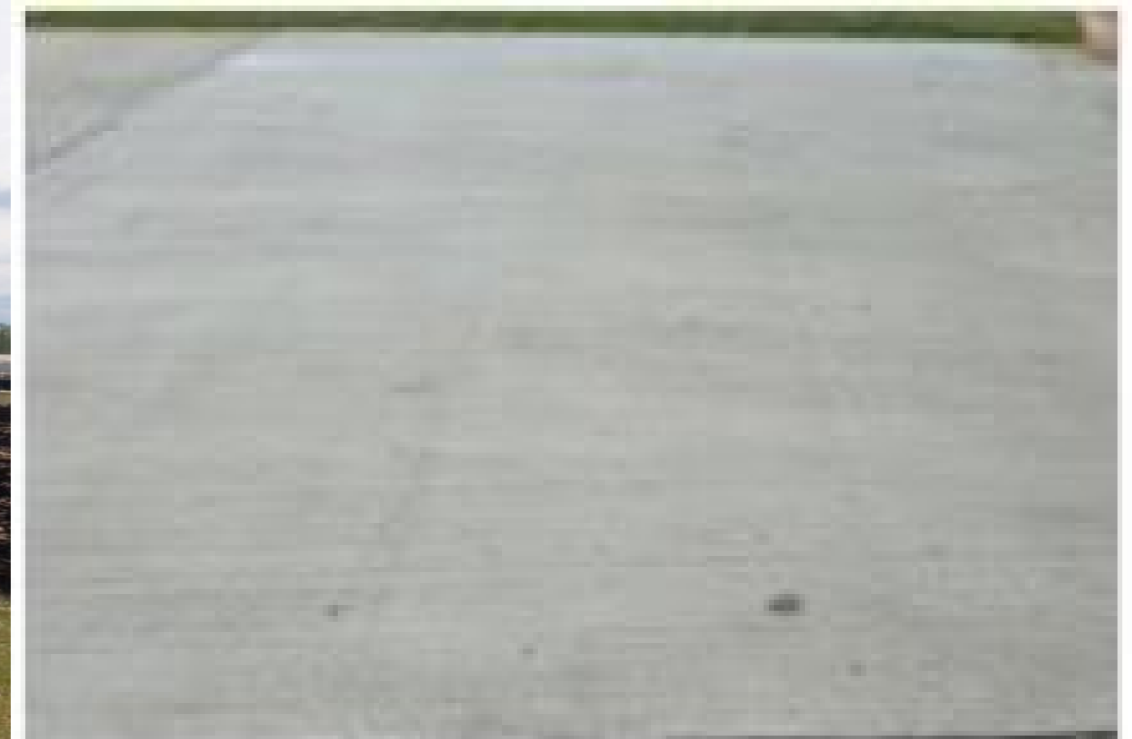
EdenCrete® TRIAL SLAB
