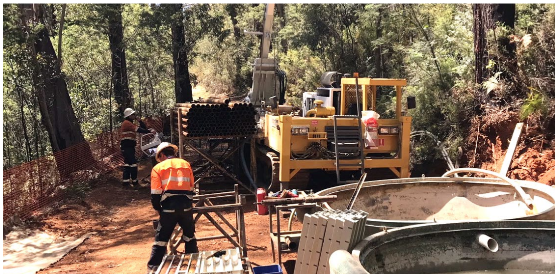
Figure 1: Diamond drilling rig on site at Hill 800.
