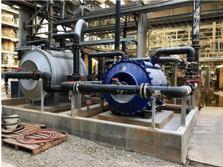
MgO Circuit Split, new heat exchangers added, new pumping designs, new hopper designs, changed filter configurations
