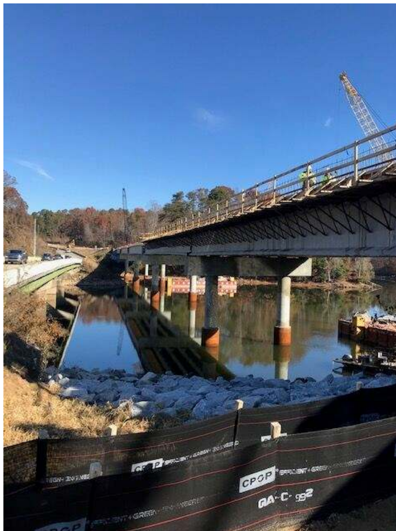
Figure 1. Bridge over the Little River
