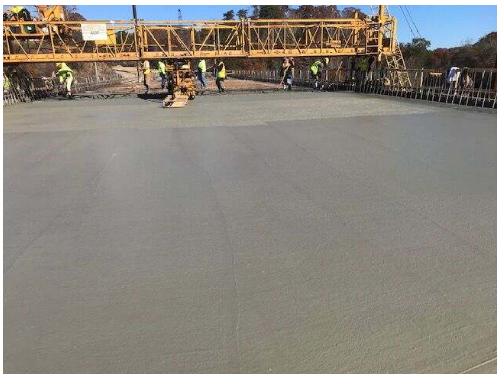
Figure 3. Bridge over Little River showing freshly lain concrete bridge decking
