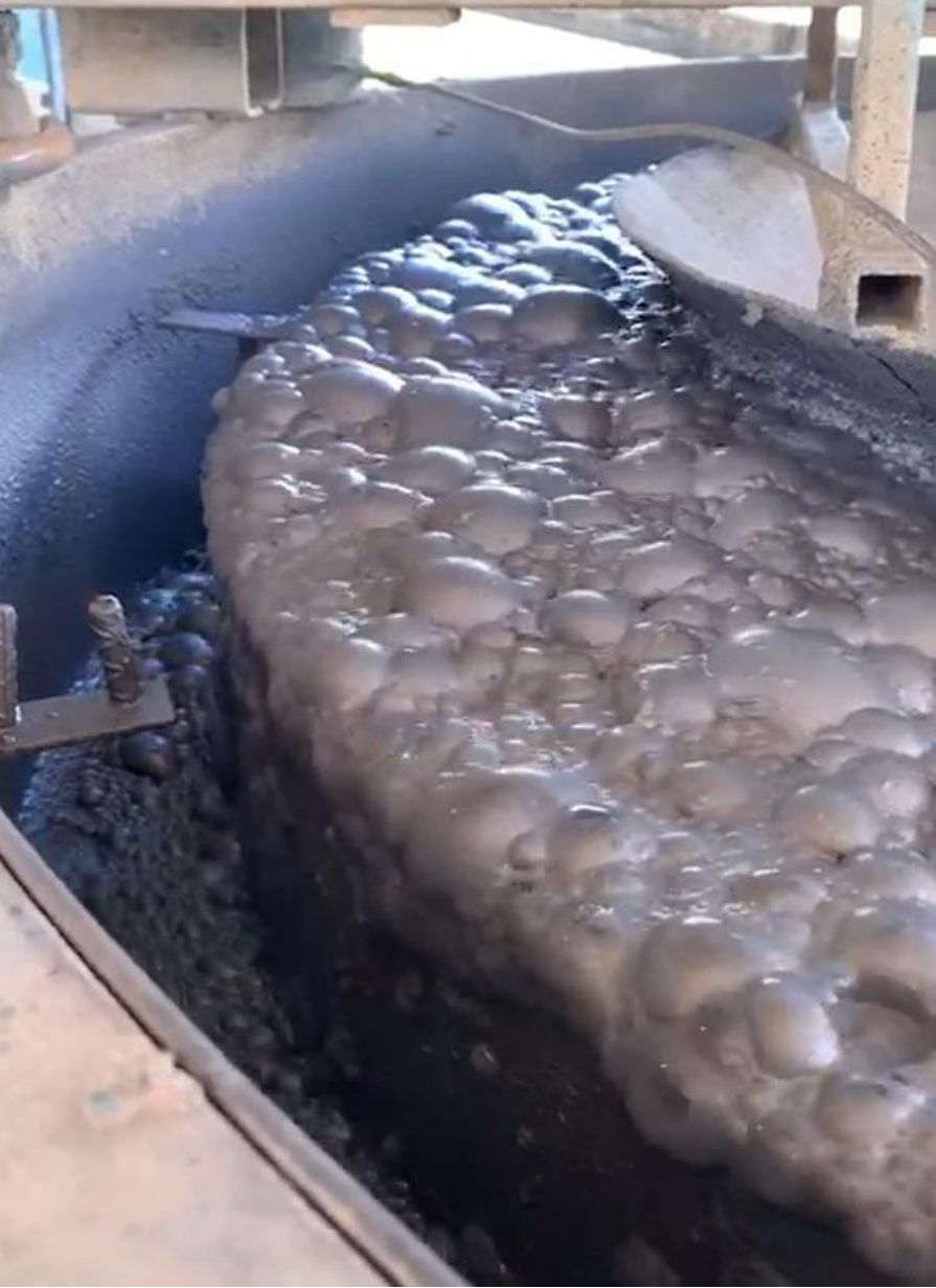
Oposura trial processing Tecoripa Plant Flash float cell #1
