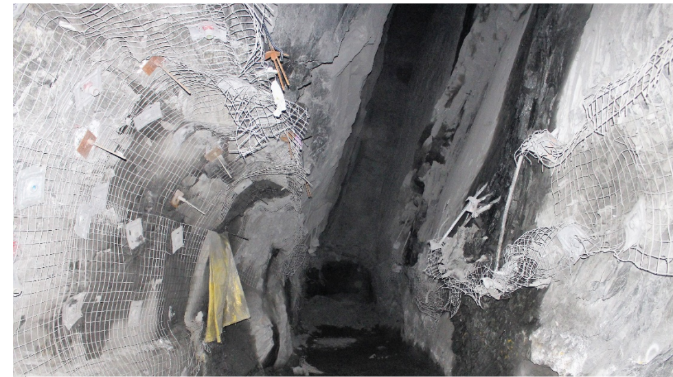
Good stoping conditions at Beresford South
