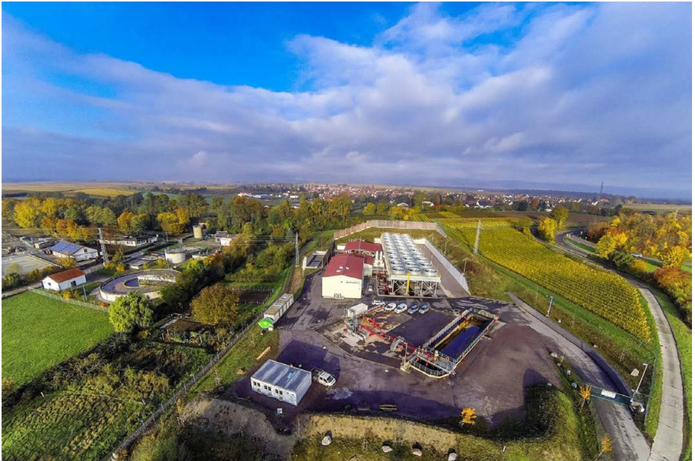
Figure 9: Insheim plant, showing harmony with local surroundings
