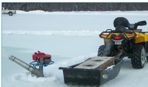
Figure 3 Thickening Lake Ice in preparation for Drill Pads
