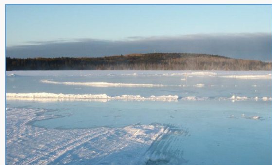
Figure 3 Thickening Lake Ice in preparation for Drill Pads
