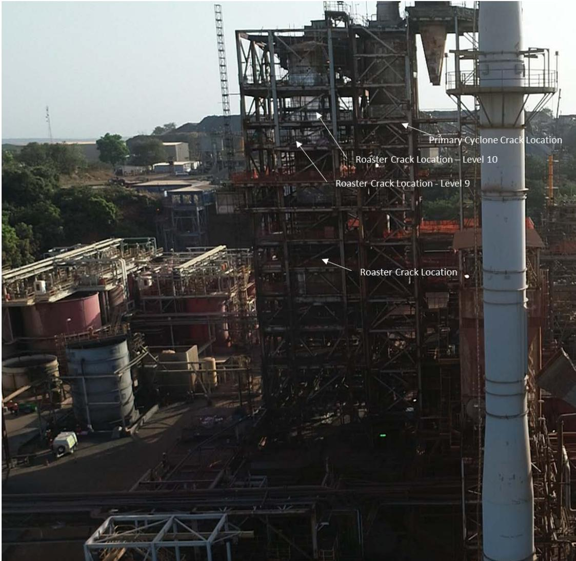
Figure 1: Syama Roaster showing repair locations
