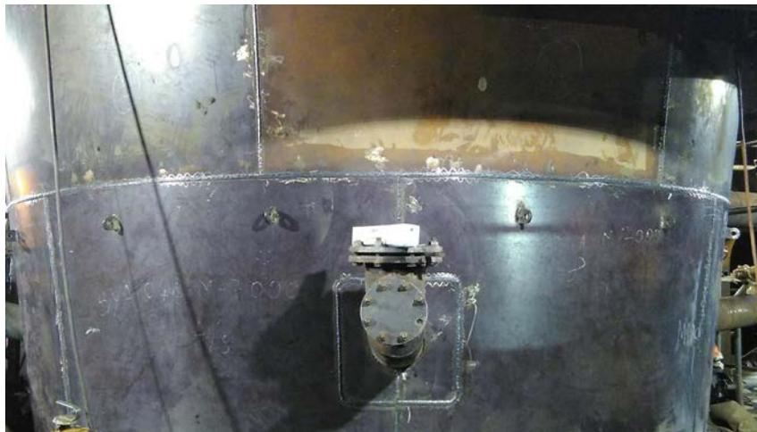
Figure 2: Syama Roaster steel replating
