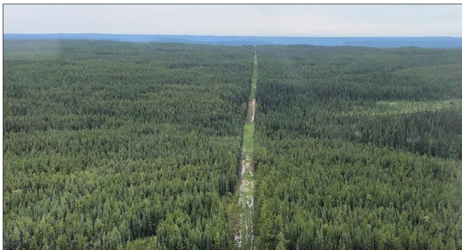
Figure Two – The proposed pipeline route through the northern part of the Calima Lands follows an existing track.
