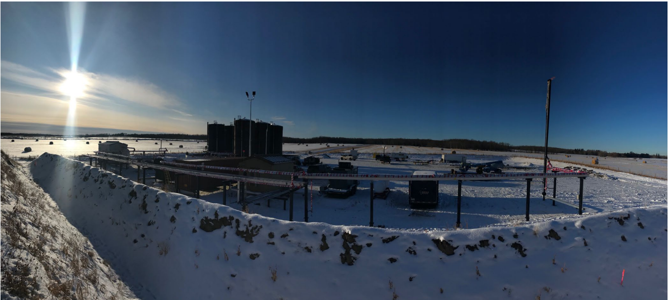
Figure 2 - Wizard Lake New Surface Facilities
