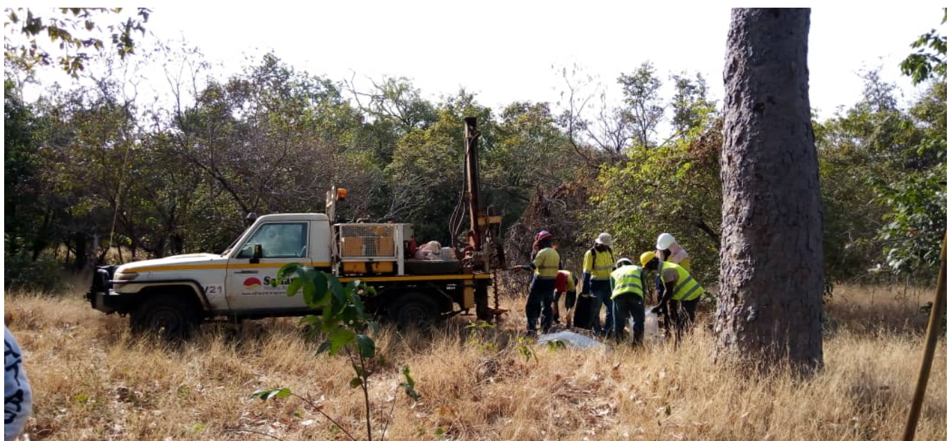
Figure 2: Drill Rig & Crew undertaking Drilling Operations
