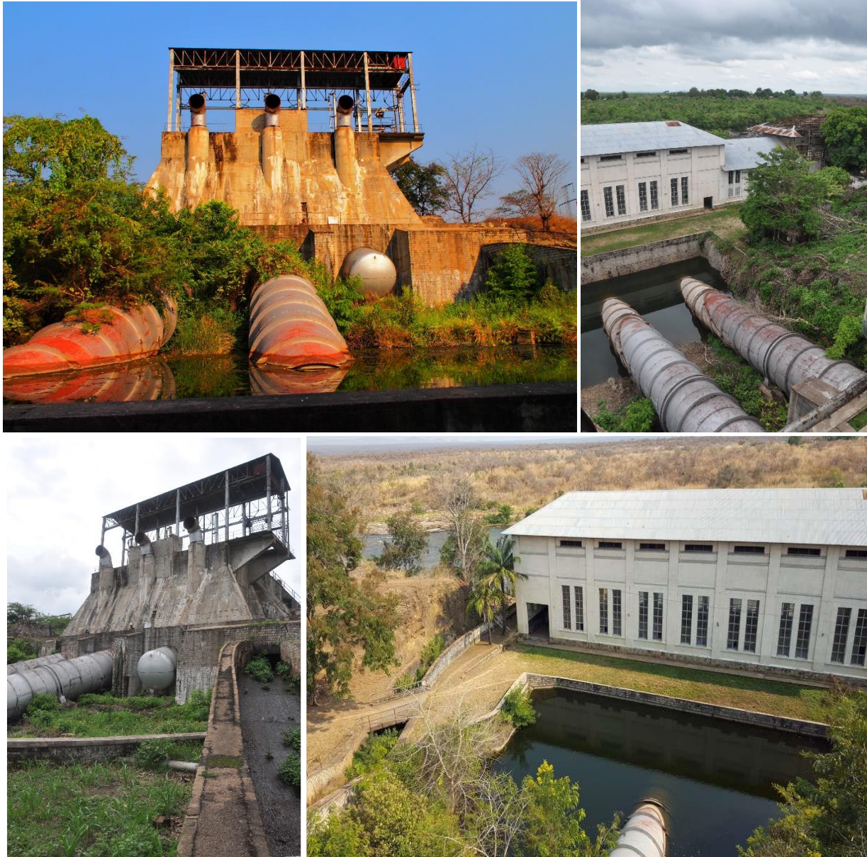
Figures 2-5: The Mpiana-Mwanga hydro-electric power station on the Luvua River
