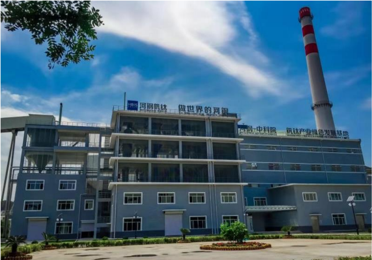
Figure 1: HBIS Vanadium Plant
