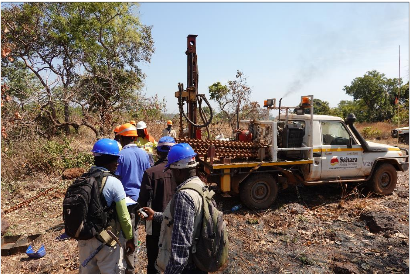
Figure 8 – Power auger drilling on the Nonta Project
