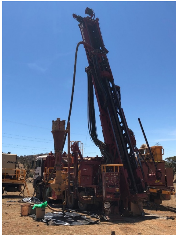
Figure 1: RC drilling recommences at Princess Royal Prospect, SA
