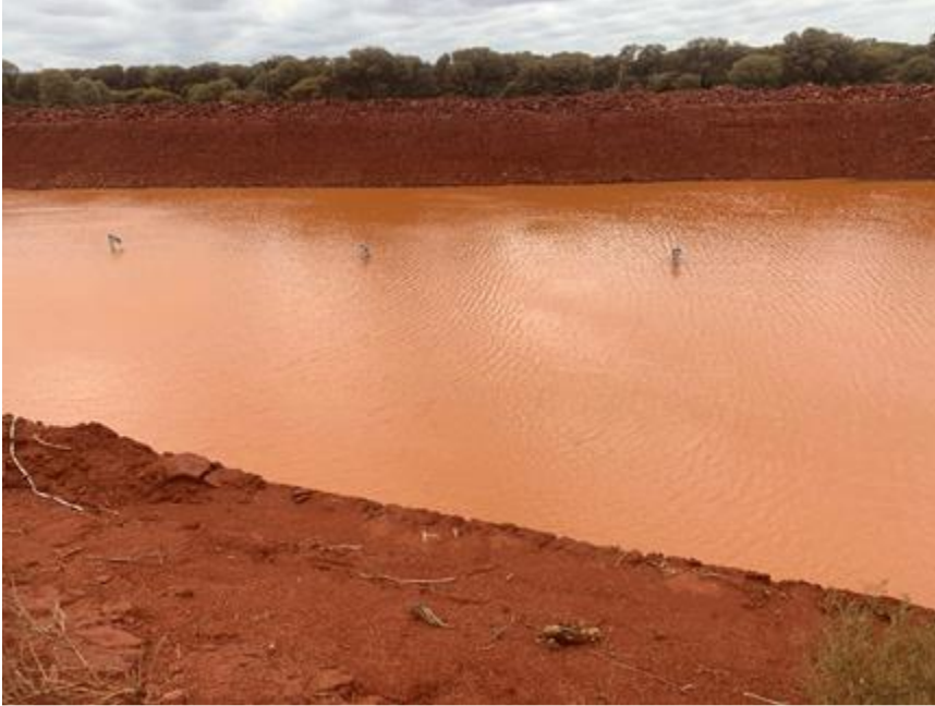
Mt Weld aquifer recharge wells after heavy rain in early January 2020, the first time with water since installation completed in 2019. The sump collects water that would otherwise run off into a nearby salt lake
