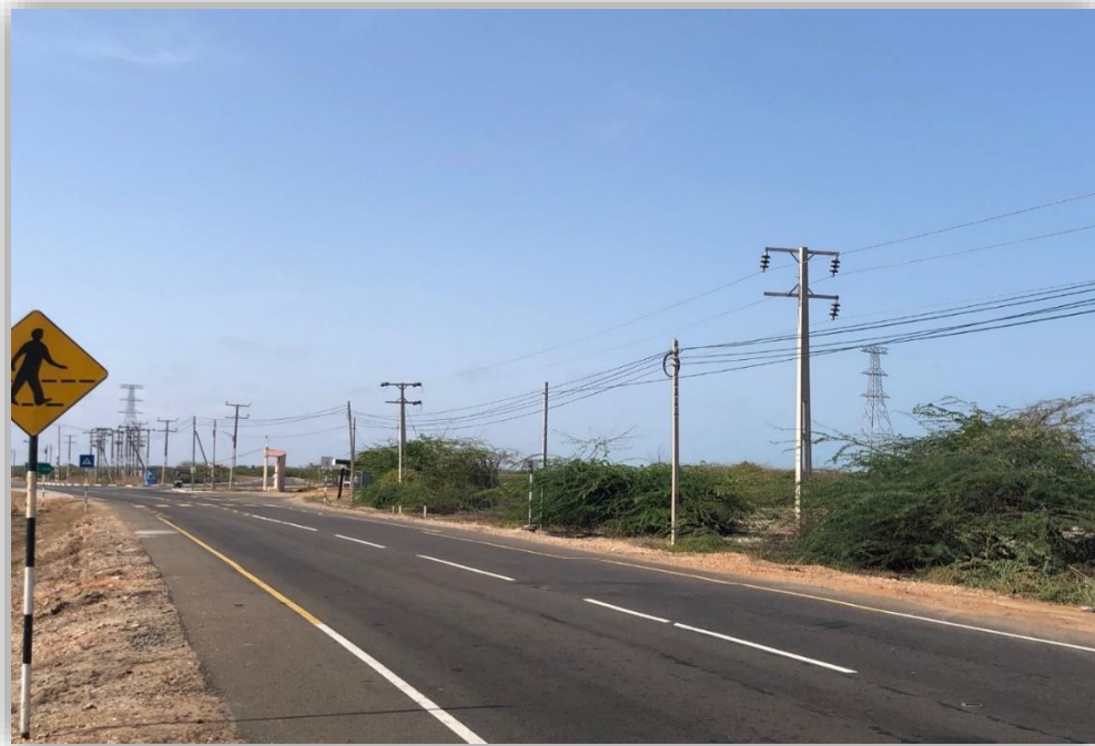
Figure 12 Road and power infrastructure leading to Mannar Island
