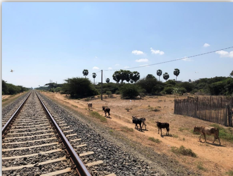
Figure 11 Rail track on Mannar Island that connects to the mainland network.
