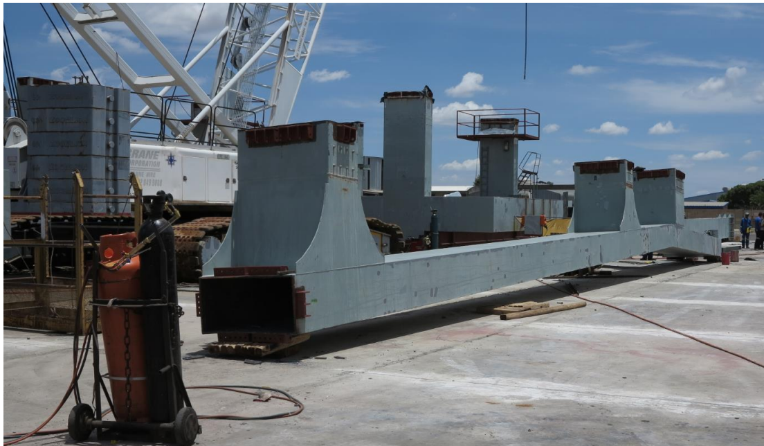
Headframe modifications in progress
