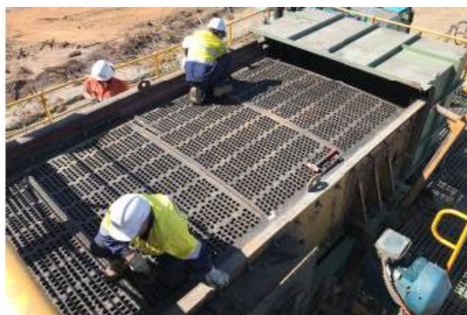
Maintenance underway on the crusher product screen
