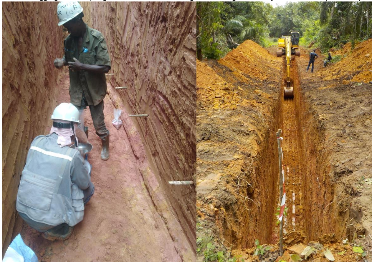
Plates 1 and 2: logging and sampling Trench 1 and excavating trench 2 Agboville Project Southern Tyche Prospect
