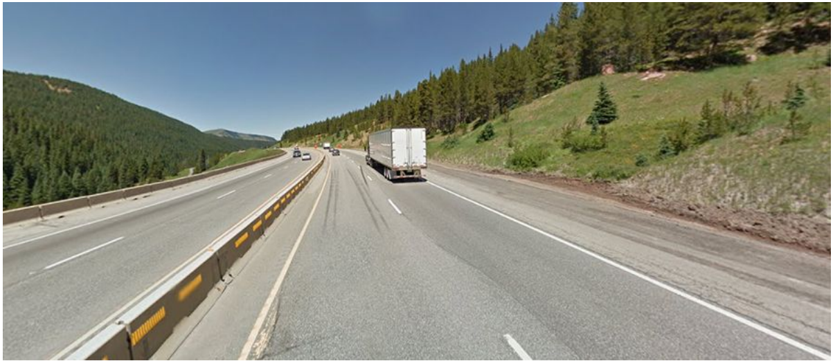
Figure 2. Interstate Highway I-70 – Vail Pass, Colorado
