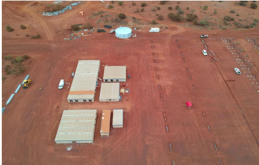
Installation of the accommodation village
