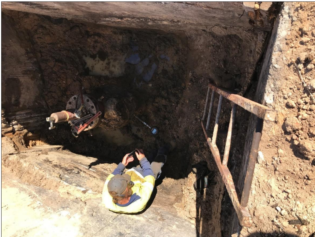
Pressure Testing Activities at Mount Horner (L7)
