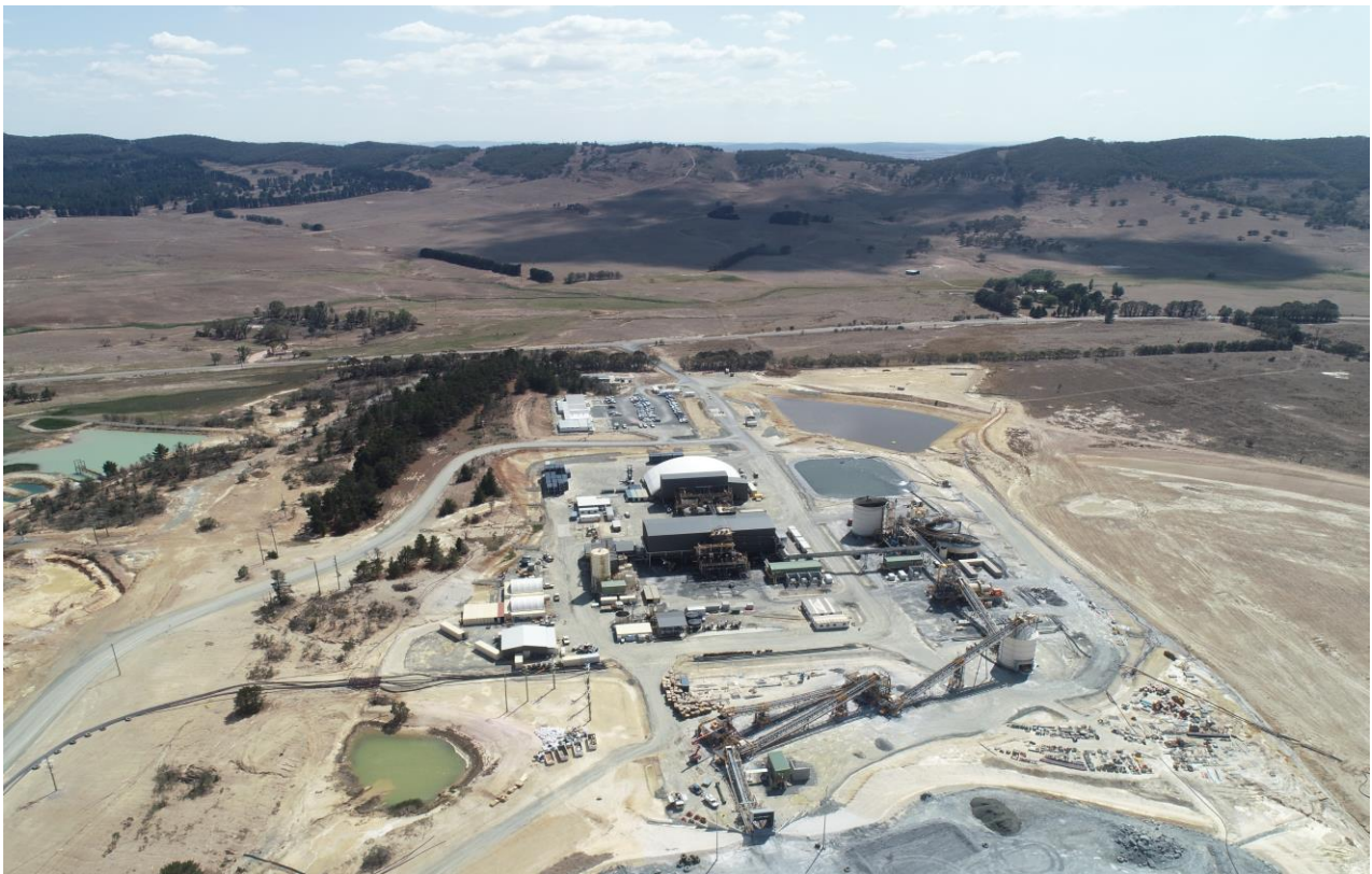
Figure 1 - Woodlawn Processing Plant, with ROM Pad, crusher and fine ore bin in the foreground
