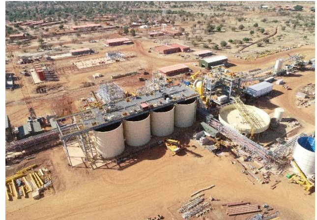
Plant area mid December 2019
