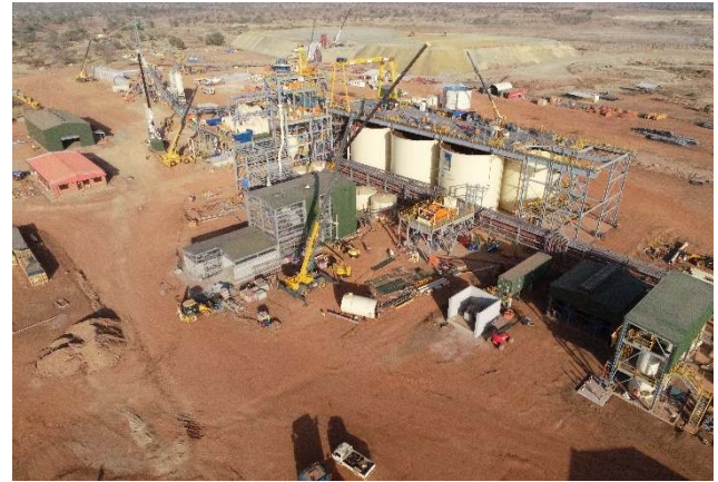
Plant area mid December 2019
