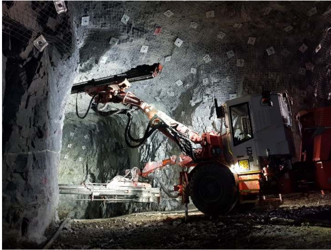
Decline being advanced at M1 South.
