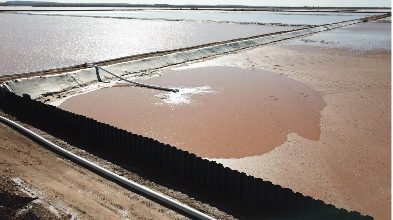
Figure 6: Commissioning of Stage 2 Evaporation Ponds
