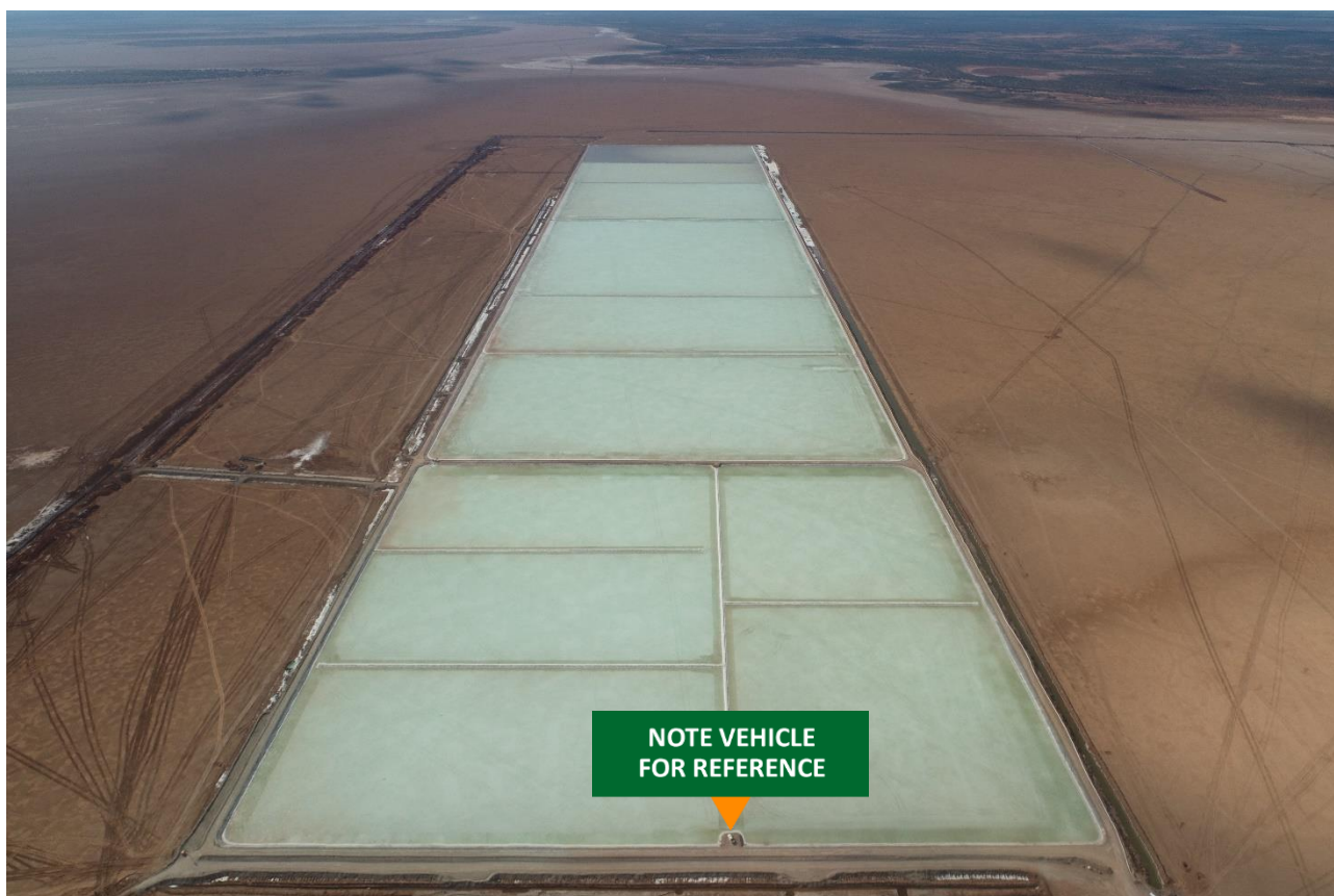
Figure 11: Completed Stage 1 solar evaporation ponds
