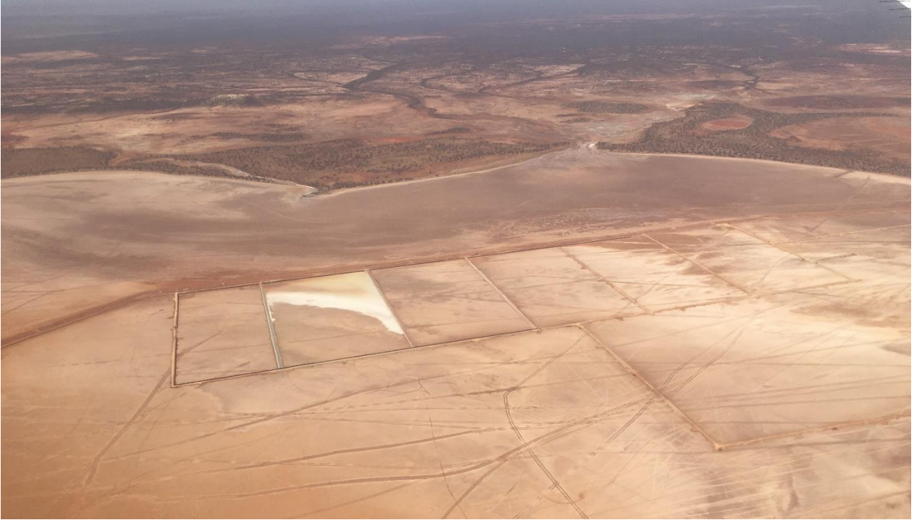
Figure 4: Aerial Photo of initial commissioning of Stage 2 Evaporation Ponds
