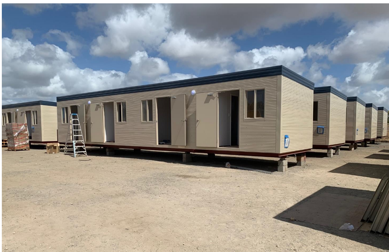
Figure 14: Manufacture of the Village Accommodation Modules Progressing
