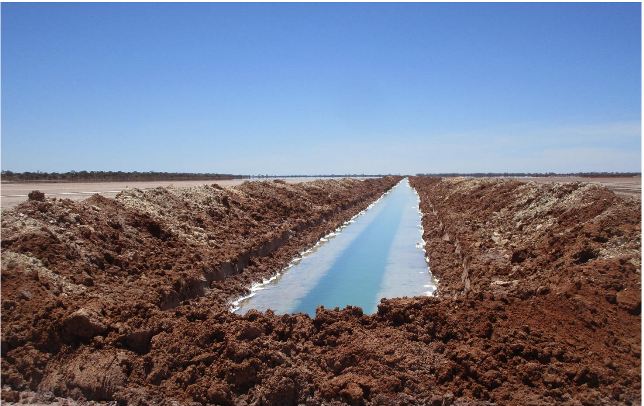
Figure 7: Stage 2 Brine Extraction Trenches
