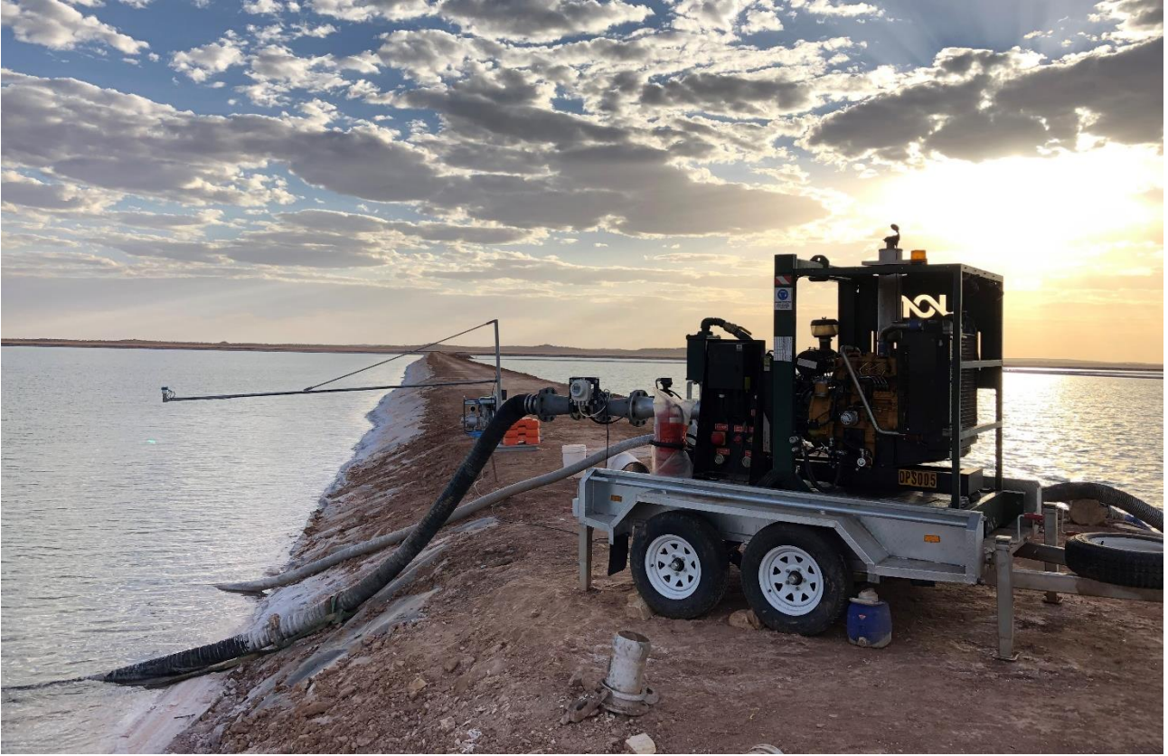
Figure 12: Commercial Stage 1 evaporation ponds in operation
