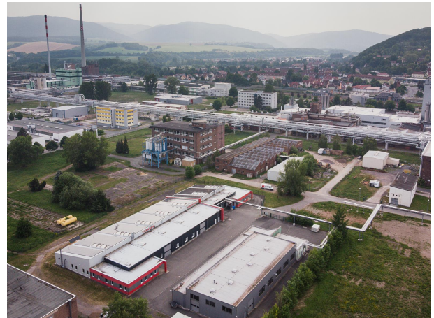
Figure 3. Talga's test processing facility in Rudolstadt, Germany.
