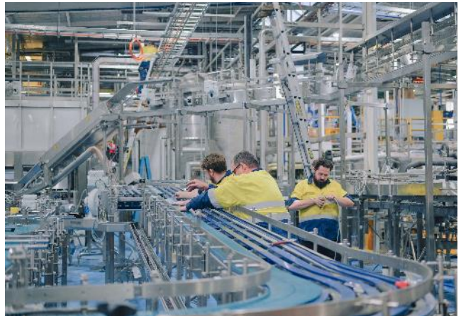
New conveyors being fitted
