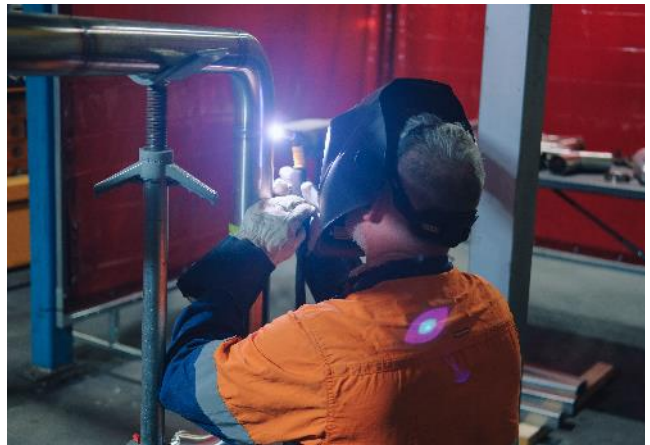
Custom pipework being assembled
