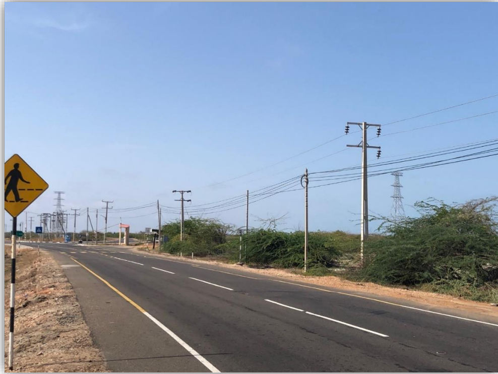
Figure 7 Road and power infrastructure leading to Mannar Island
