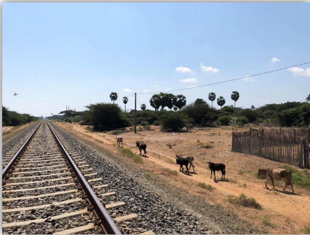
Figure 6 Rail track on Mannar Island that connects to the mainland network.
