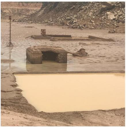
Figure 3 – The sump on the floor of the Roche Dure pit, post dewatering
