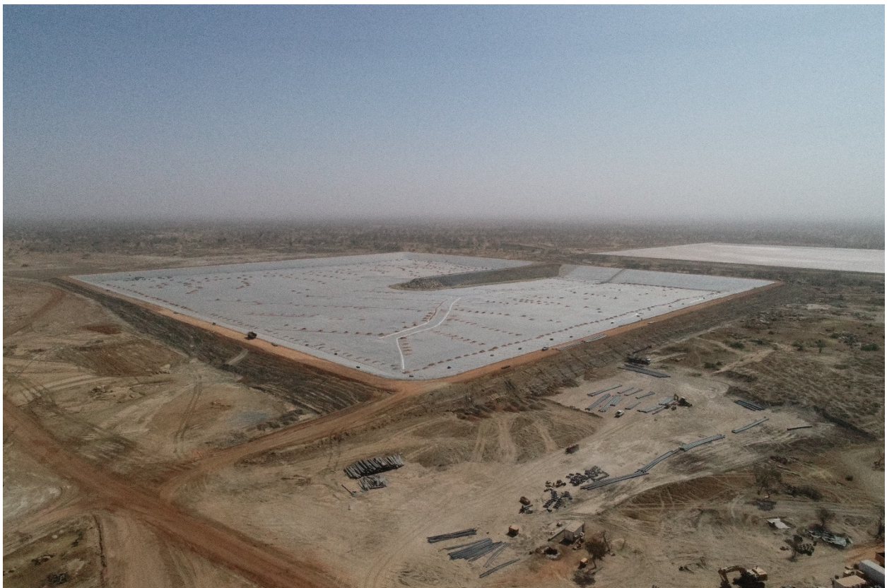
Photo 5: Completed HDPE lined tailings facility, and water storage dam in distance [POD: crop]
