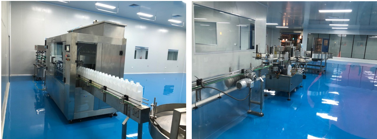
Newly installed bottling line at Mill Park
