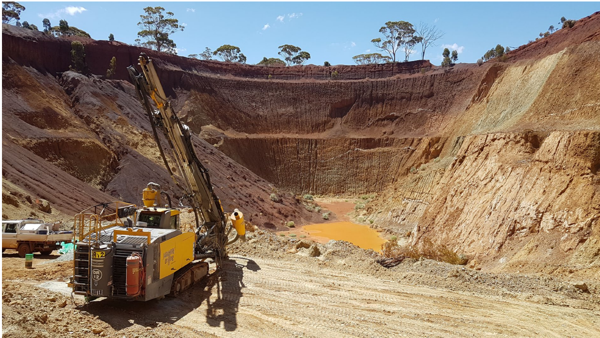
Drilling at Panther Pit 14 February 2020
