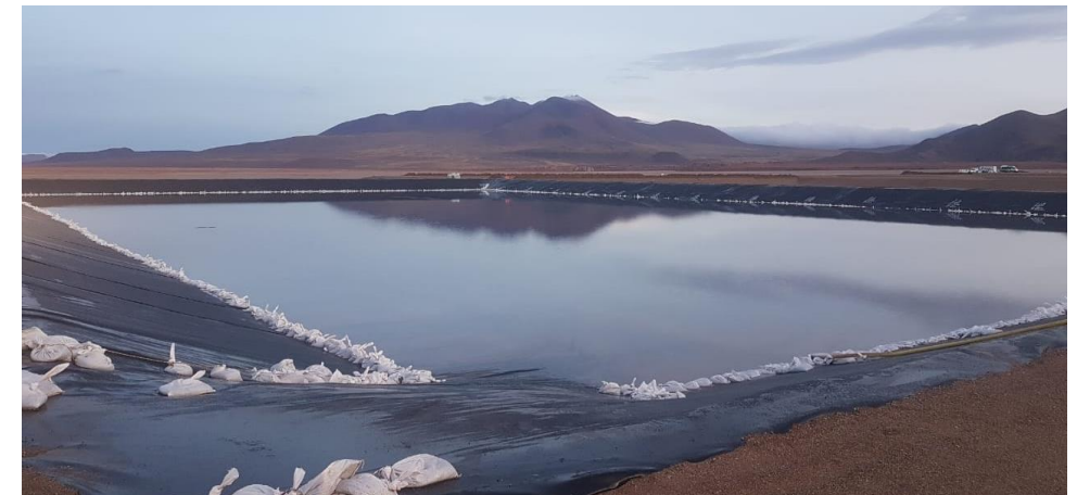
Ponds are well advanced with lining and filling underway
