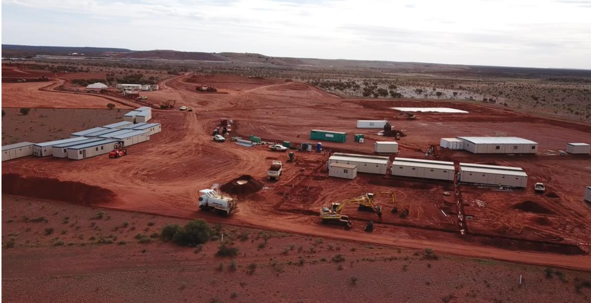
Figure 11: Early stage civils at processing plant site
