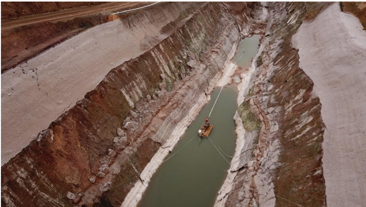
Figure 10: Williamson Pit de-watering nearing completion
