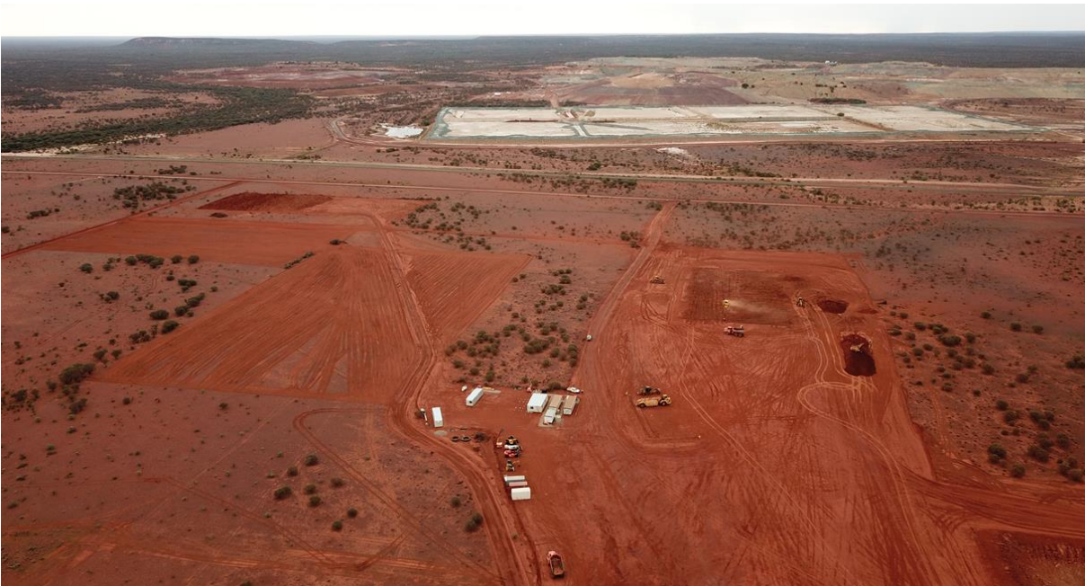
Figure 12: Early stage civils at processing plant and village site
