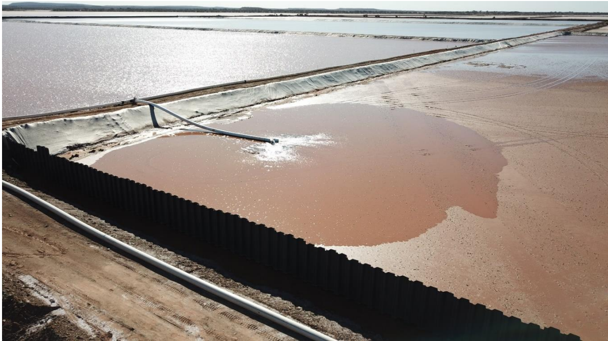
Figure 1: Stage 2 pond filling with brine
