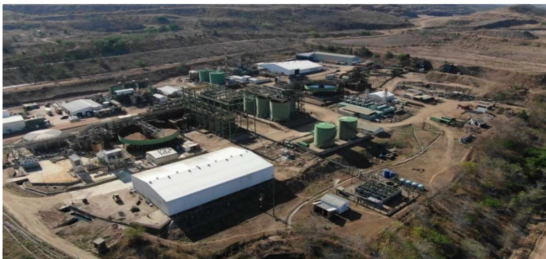
Figure 1 - More than $200M was invested into infrastructure at Kayelekera uranium project, which was in production from 2009 to 2014
