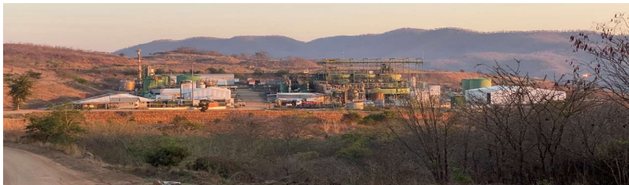
Figure 2: Kayelekera Process Plant and Surrounds – October 2019
