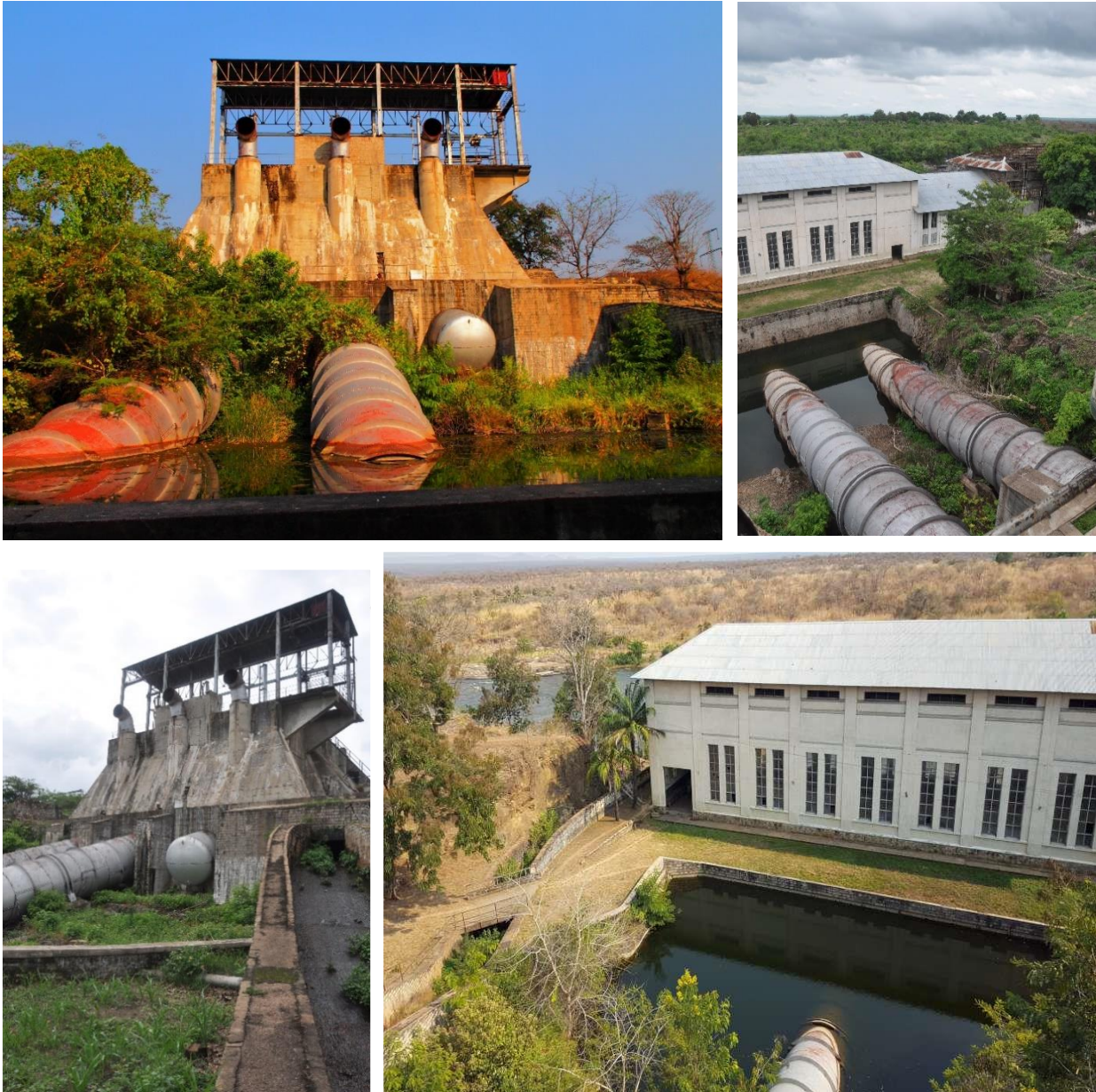
Figures 4-7: The Mpiana-Mwanga hydro-electric power station on the Luvua River
