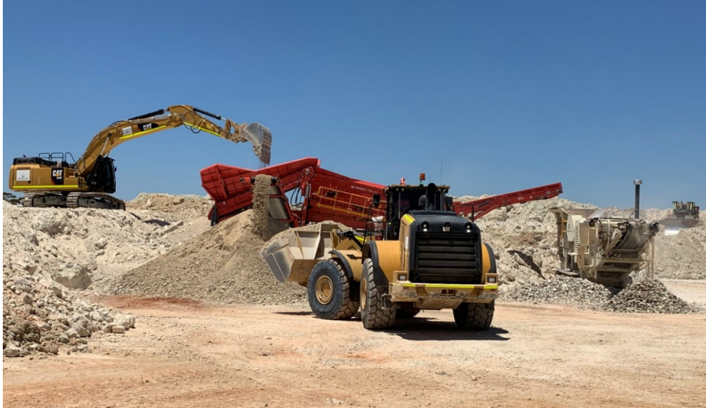
Figure 2 – Screening and Crushing on the Jaurdi ROM pad
