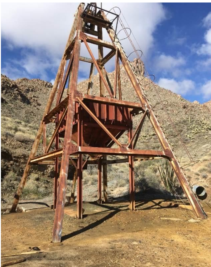
Headframe at the Antler Copper Mine
