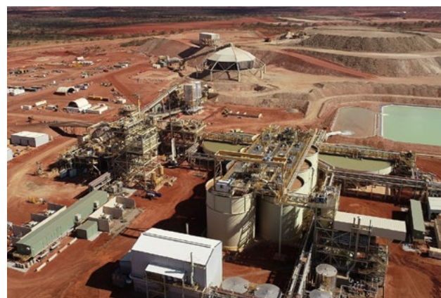
Aerial view of Gruyere Process Plant
