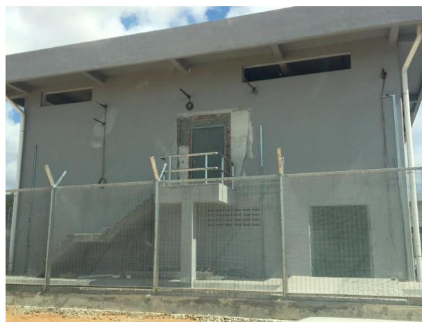
Figure 2 – Completed substation structure, fenced
