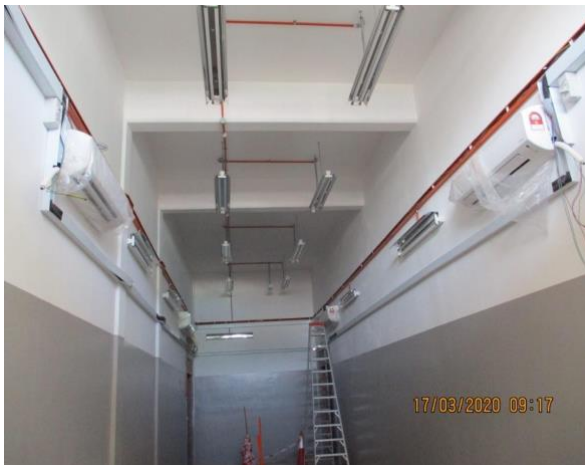
Figure 1 – Substation internal finishing
